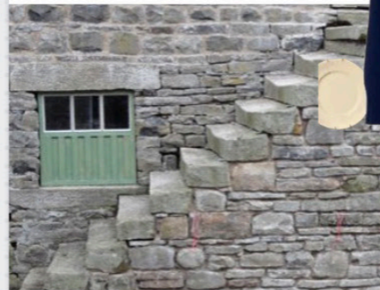
Continuing to move through the space..
